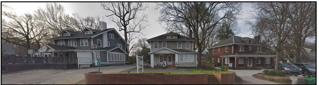
The properties to the south along North Caswell Road are developed with a mix of office, retail and an EDEE.
