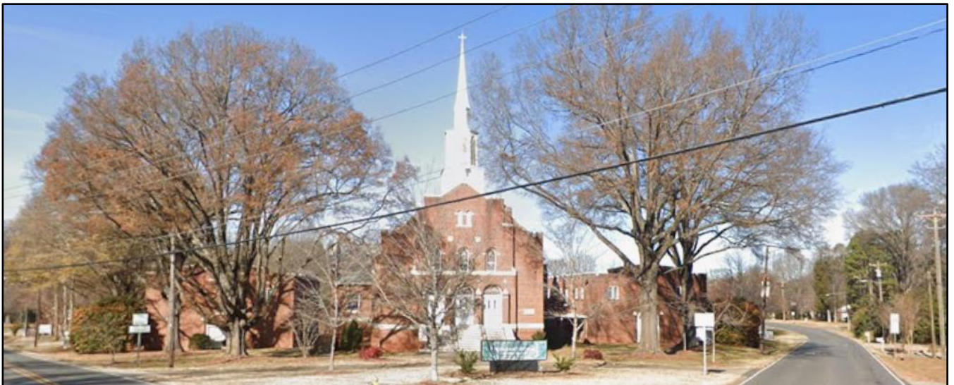
View of a church located northwest of the site at the intersection of Oakdale Road and Pleasant Grove Road.
