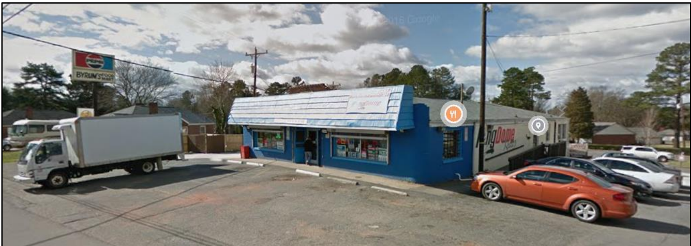
View of a commercial development located across Oakdale Road to the west of the subject site zoned CG (General Commercial). The development contains retail, restaurant, and personal services uses like a barber shop.
