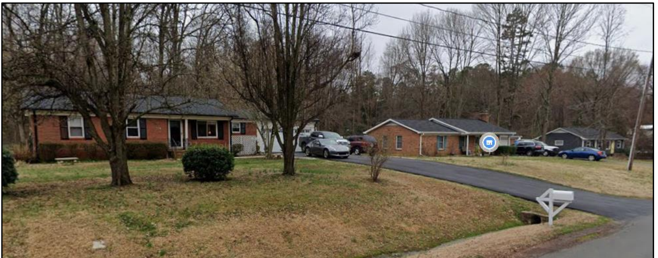
View of single family houses along Ravendale Drive south of the site. The houses are on lots typical of the development pattern in the area, approximately 90 feet in width with an area of approximately 15,000 square feet.
