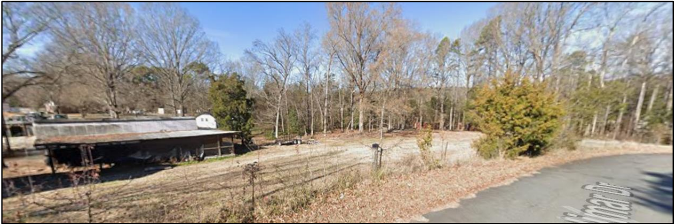
View of the site looking west from Shalimar Drive. The site is developed with a single family house and an accessory structure.
