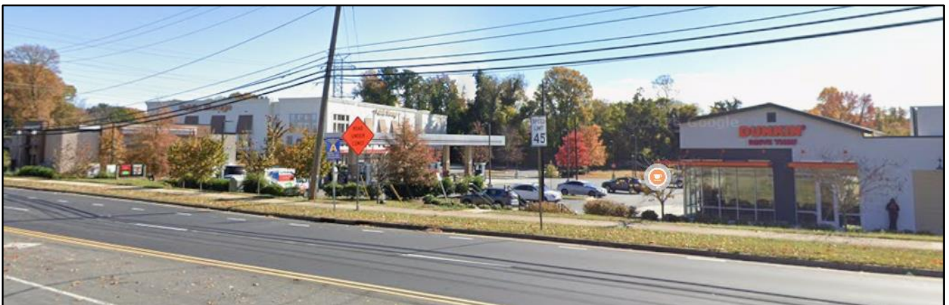
View of a small commercial development at the intersection of West Tyvola Road and South Tryon Street, abutting the property to the north. The development contains a drive-through coffee shop, gas station, and self-storage facility.
