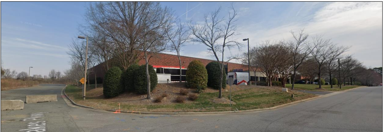
East of the site is an industrial building with some office space.
