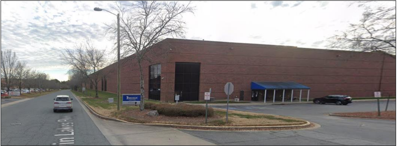
South of the site are warehouses and office space.
