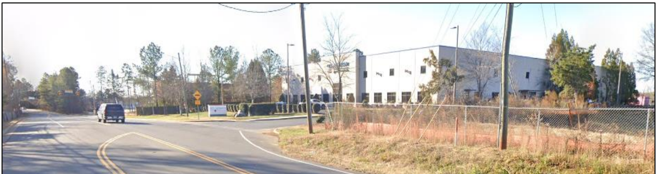
Street view of commercial and industrial uses to the east of the site along Beam Road.
