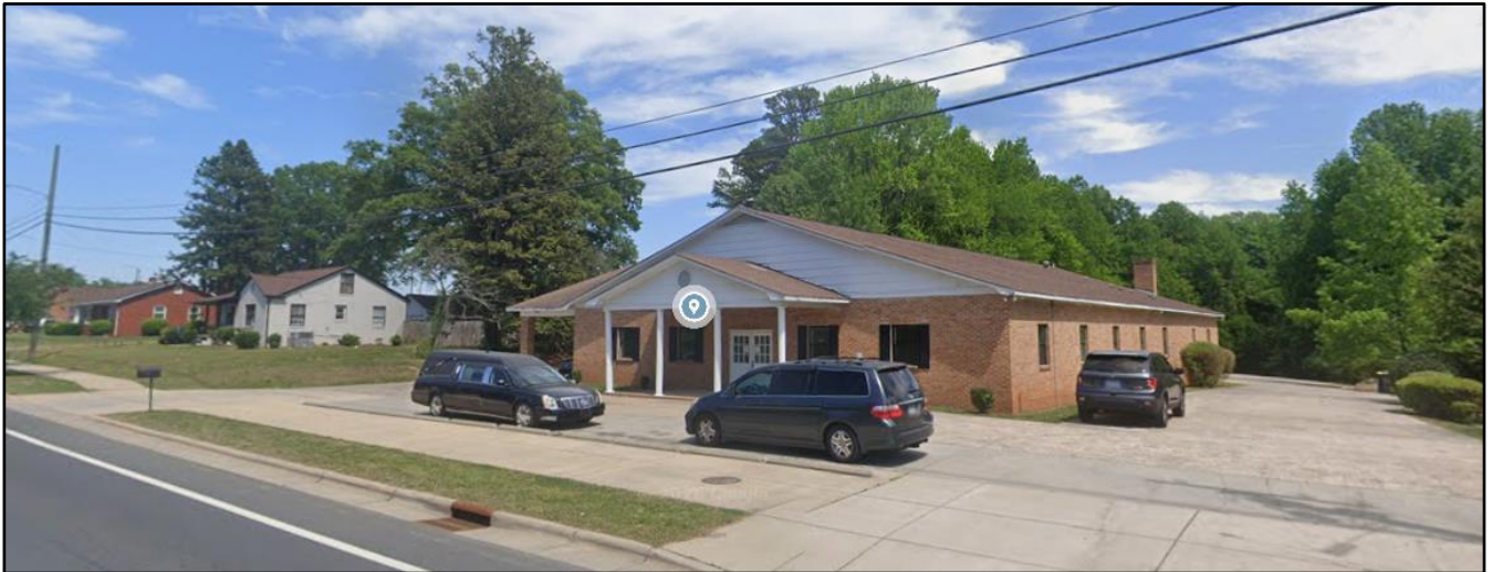
View of an institutional use abutting the subject site to the north zoned OFC (Office Flex Campus).
