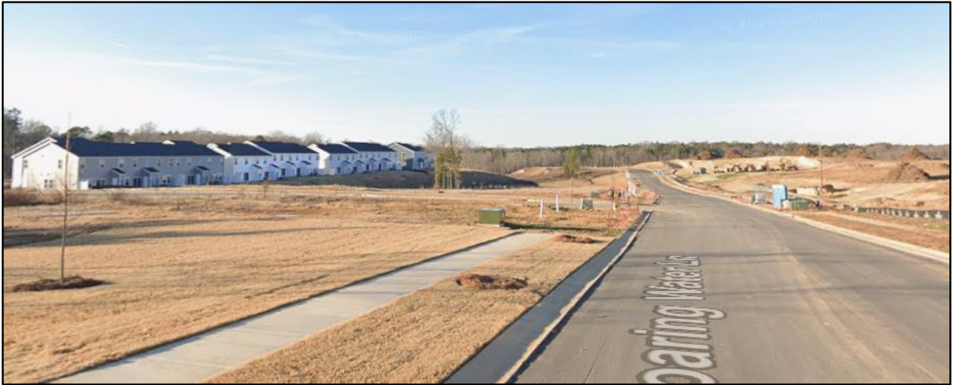
View of the multi-family attached subdivision zoned MX-2 INNOV (Mixed-Use Innovative, conditional) located across Kelly Road. The subdivision is currently under construction.
