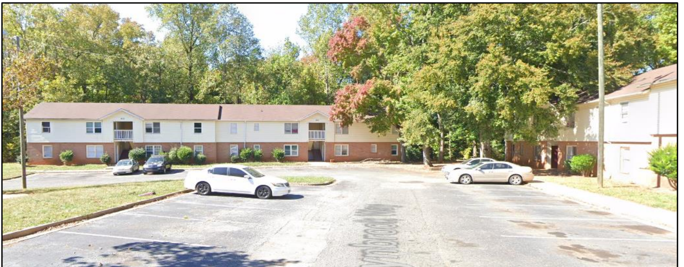
View of a the Dalecrest Multi-family development located to the east of the site zoned N2-B (Neighborhood 2-B).
