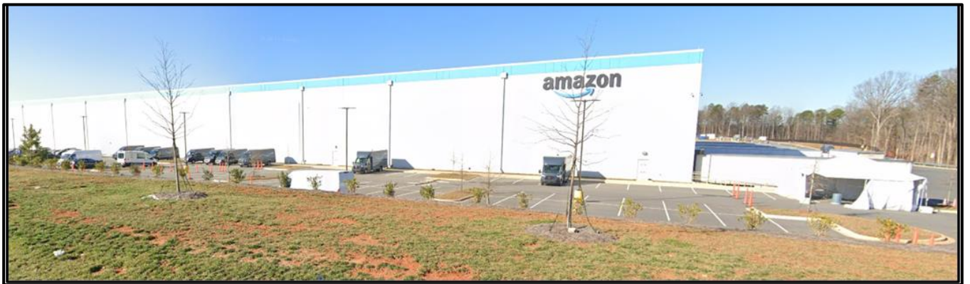
The property to the south along Old Statesville Road is the Amazon distribution center.
