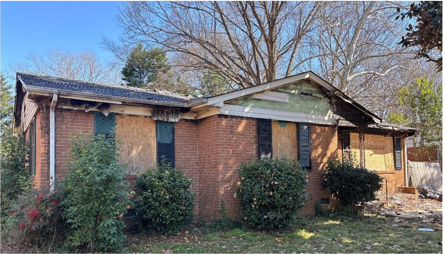
Front exterior of dwelling
