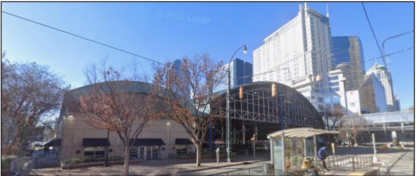
View of the Charlotte Transportation Center (CTC) looking west from East Trade Street. The CTC provides access to the subject site via bus and the LYNX Blue and Gold lines.
