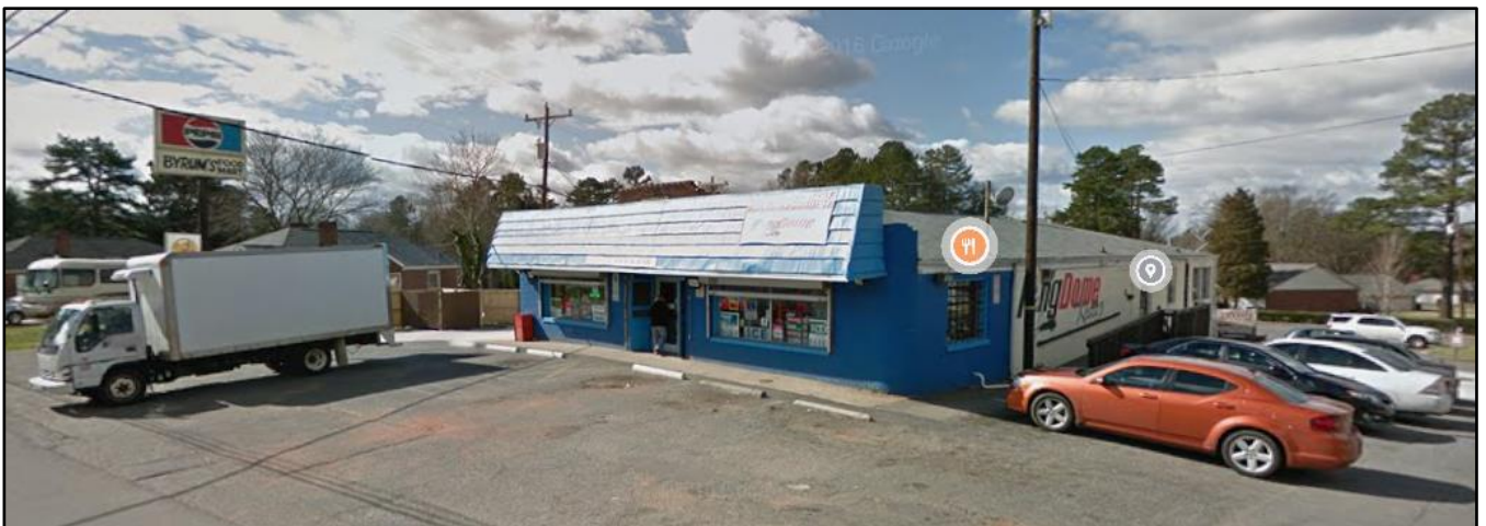
View of a commercial development located across Oakdale Road to the west of the subject site zoned CG (General Commercial). The development contains retail, restaurant, and personal services uses like a barber shop.
