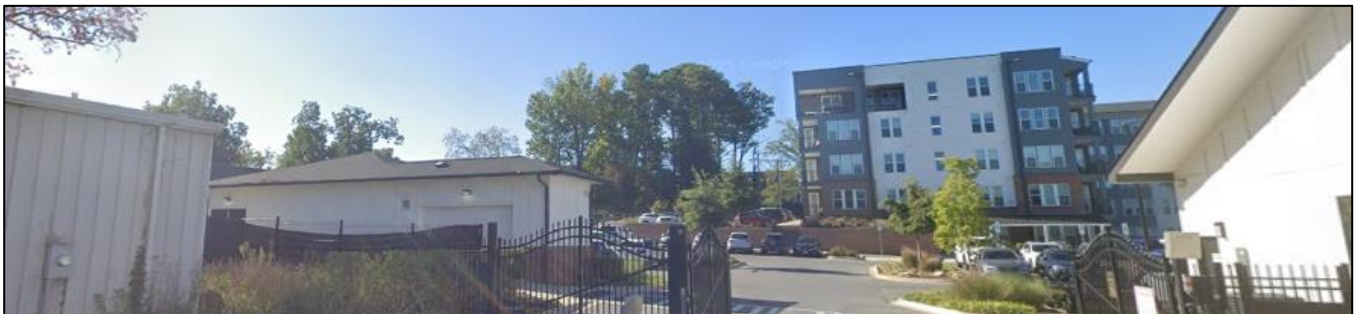
Street view of apartments to the south of the site, accessed from Verbena Street.
