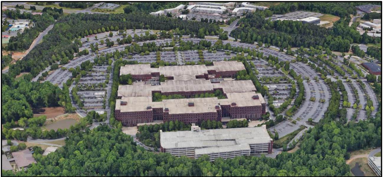
The property to the north along IBM Drive is the Wells Fargo Customer Information Center.
