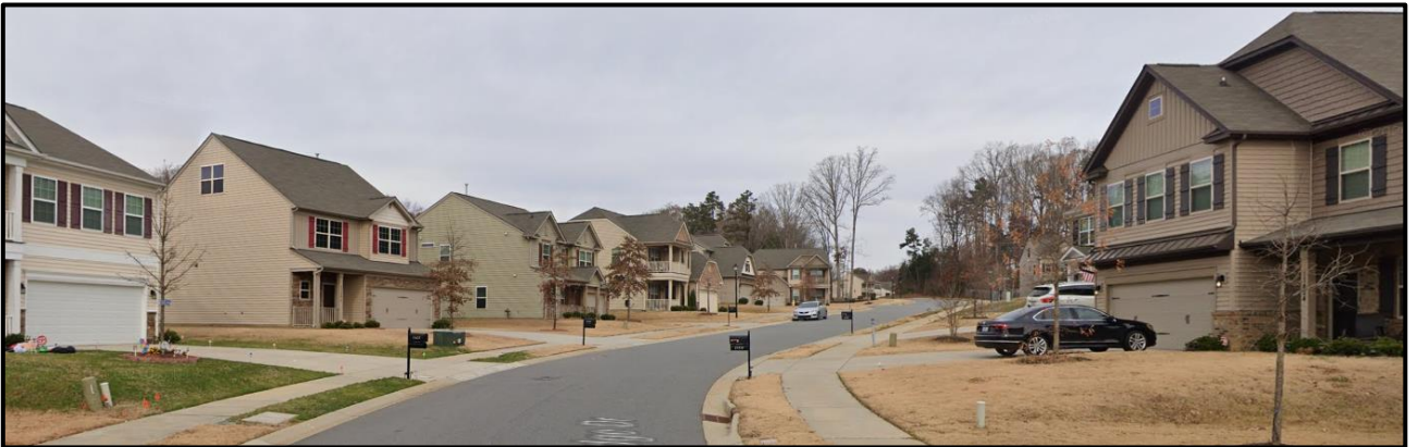
The property to the west along Sweetbriar Ridge Drive is developed with single family homes.
