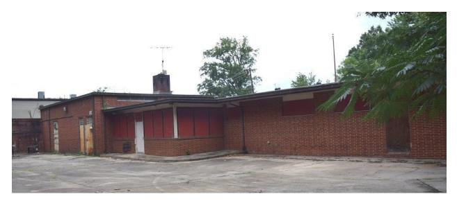
The tripart design of the fire station's facade is reflected on the rear. The northern portion of the rear elevation is five bays wide, and is sheltered by a deep eave. It is pierced by one two-light window and one set of paired two-light windows set high in the wall. The other bays contain a single-light aluminum door flanked by tripled two-light windows set high in the wall. The brick is laid in common bond with coursed Flemish headers.
