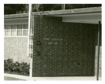
A double-wythe, blank brick wall composed of Norman brick laid in common bond with coursed Flemish headers forms the northern wall of the recessed porch and extends 16" past the roof eave. A metal flagpole is attached to the narrow edge of the projecting wall with three circular brackets.
