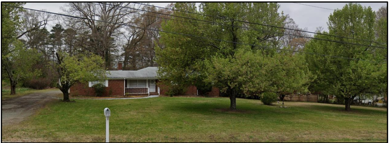
The property to the north along Reames Road is developed with single family homes.
