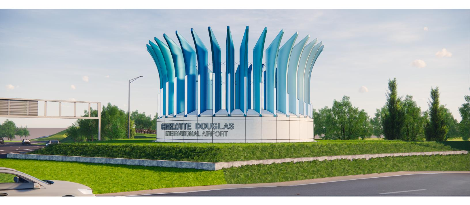
"Entry Monument": A cast-in place concrete structure with Glass Fiber Reinforced Plastic panels illuminated custom metal fins and entry signage for Charlotte Douglas International Airport
