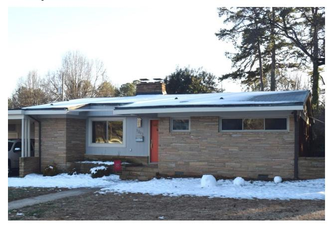
The low-pitched roof is topped with a short stone chimney, and features integrated gutters. The sandstone found on the façade extends uninterrupted to the west as a partial-height wall.
