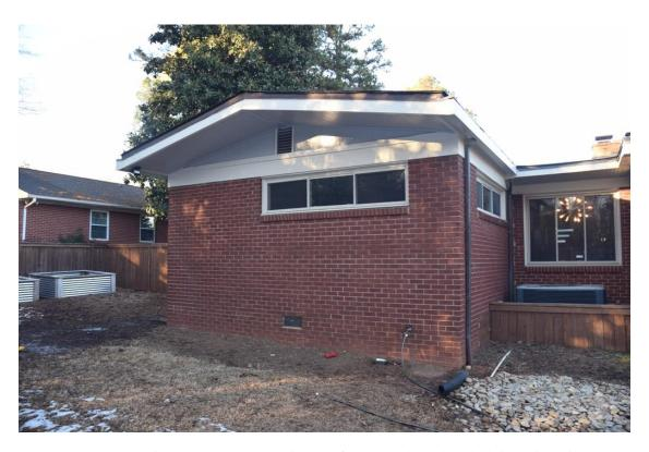
The asymmetrical rear elevation of the gabled addition is pierced by a tripart sliding windows set high in the wall and resting on an angled brick sill. The wall is topped with a wide simple band. The low-pitched roof features a deep overhang. The gable is sheathed with T1-11 and features a center louvered vent.
