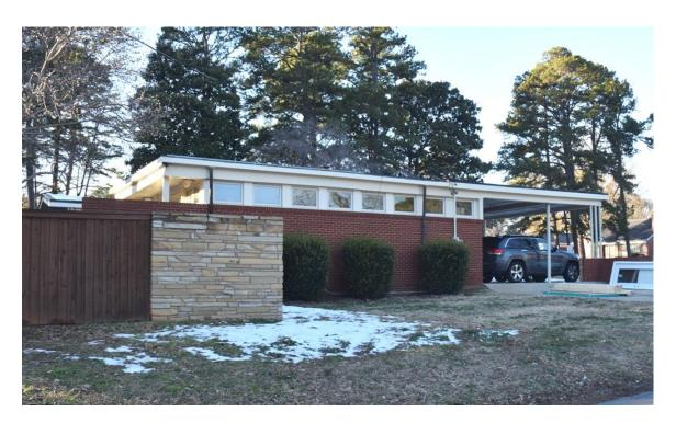
The carport is engaged with the flat-roofed wing, which extends past the rear elevation of the principal section of the house. The east elevation of the wing is composed of a blank, partial-height brick wall topped with a full-width, eight-sash ribbon window.
