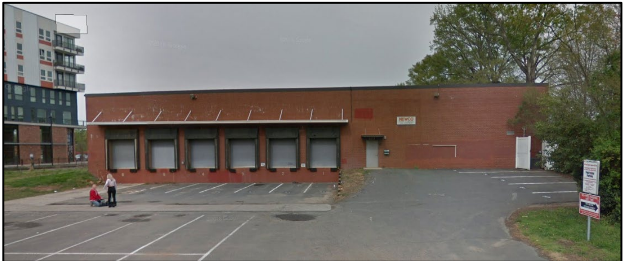
The subject property is developed with a warehouse use.
