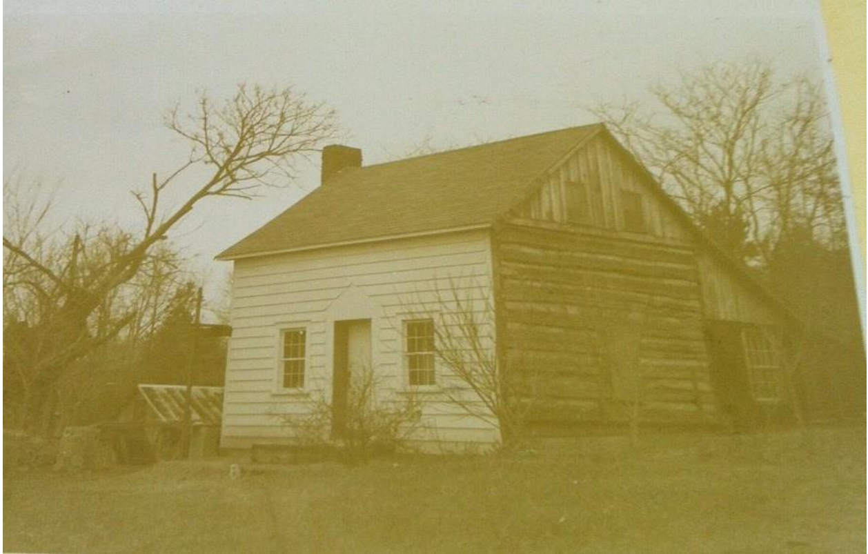
A 1950 photograph shows the front elevation covered with lap siding. A new window has been cut into the front elevation to the east of the door. The east elevation features exposed logs with a window centered on the wall. The gable is covered with vertical board-and-batten siding. Two small windows are set in the gable. The roof has a minimal overhang. The roof extends to the rear to cover a one-bay-deep, frame addition with a large double-hung window set in the east elevation of the addition.
