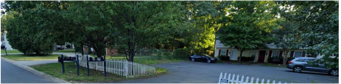
Street view of the site from Mayfair Avenue showing one single family detached dwelling and a quadrplex building.
