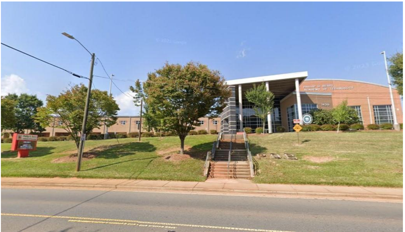
View of the Philip O. Berry Academy of Technology located on Alleghany Street northeast of the site. There are three schools located with a ½-mile walking distance of the site including Harding University High School and Ashley Park Elementary School.
