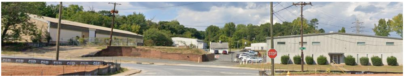
Street view of industrial uses that currently occupy the site.
