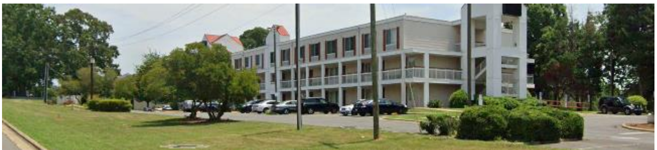
Streetview of hotel use to the south of the site across Queen City Drive. The properties to the east and west of the site are also developed with hotel uses.
