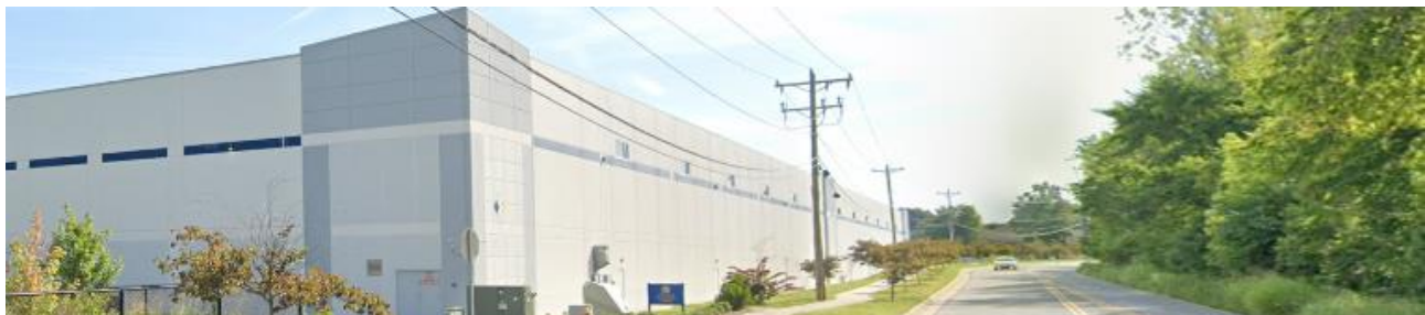
Streetview of industrial uses north of the site across John Price Road.
