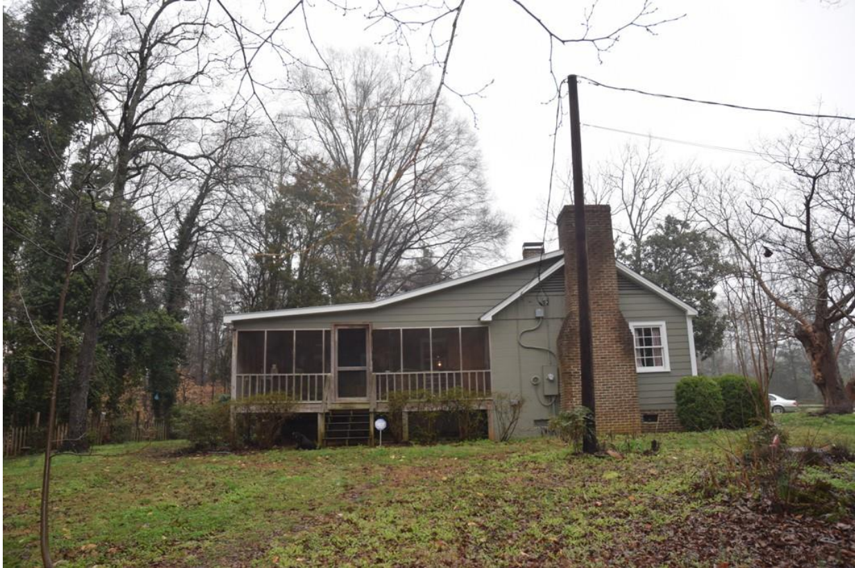
A two-part shed roof extends from the rear of the block wing, and covers a screened porch that is supported by wooden posts.
