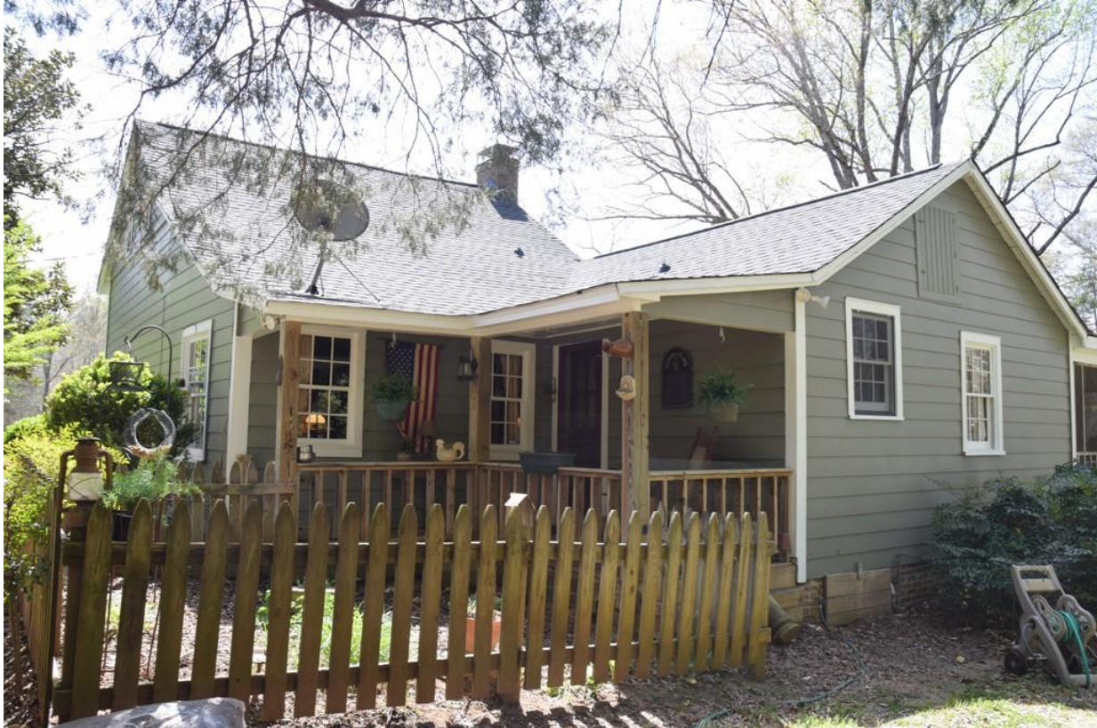
A shed-roofed porch and a ca. 1956 gabled wing extend from the rear of the house. The rear wing rests on a brick foundation.
