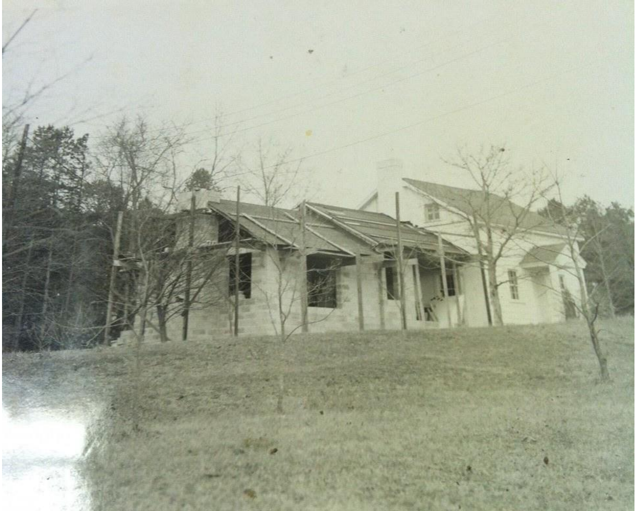
A ca. 1956 photograph shows a block (CMU) wing being constructed on the west elevation. The principal section of the house features a small gabled porch supported by boxed posts. The west elevation is covered with siding. The façade features a replacement vertical-board door. The windows on the facade are flanked by simple decorative shutters.
