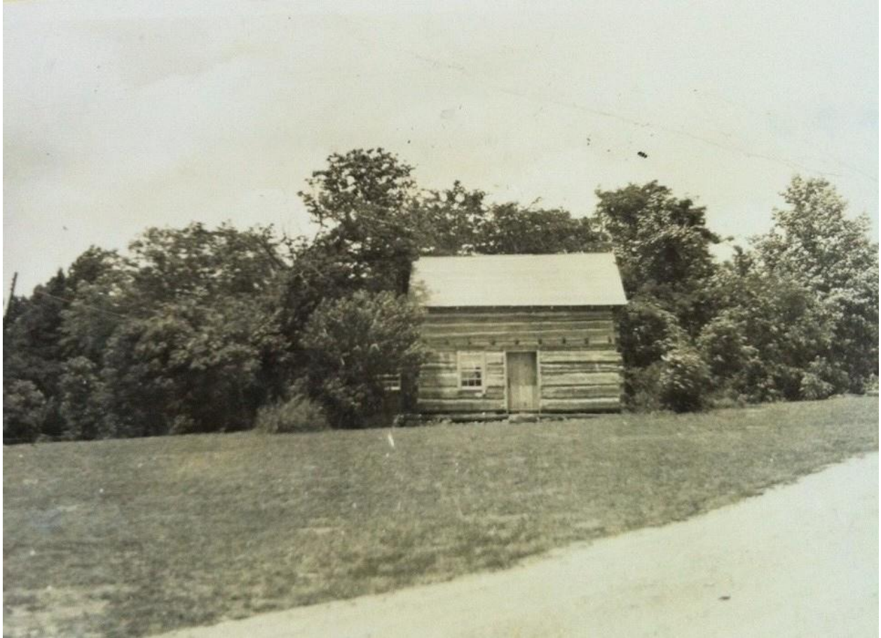
A 1949 photograph shows a restored log house, with exposed chinking, and repaired or replaced windows. The log house features a door centered in the façade. Originally additional fenestration on the façade was limited to a single window to the west of the door. The west elevation features a centered, shouldered, brick chimney.
