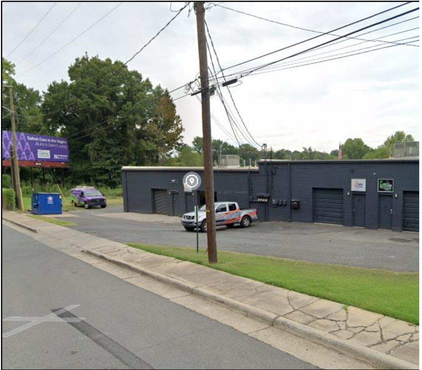
The property to the south along West Tremont Avenue is developed with a commercial use.
