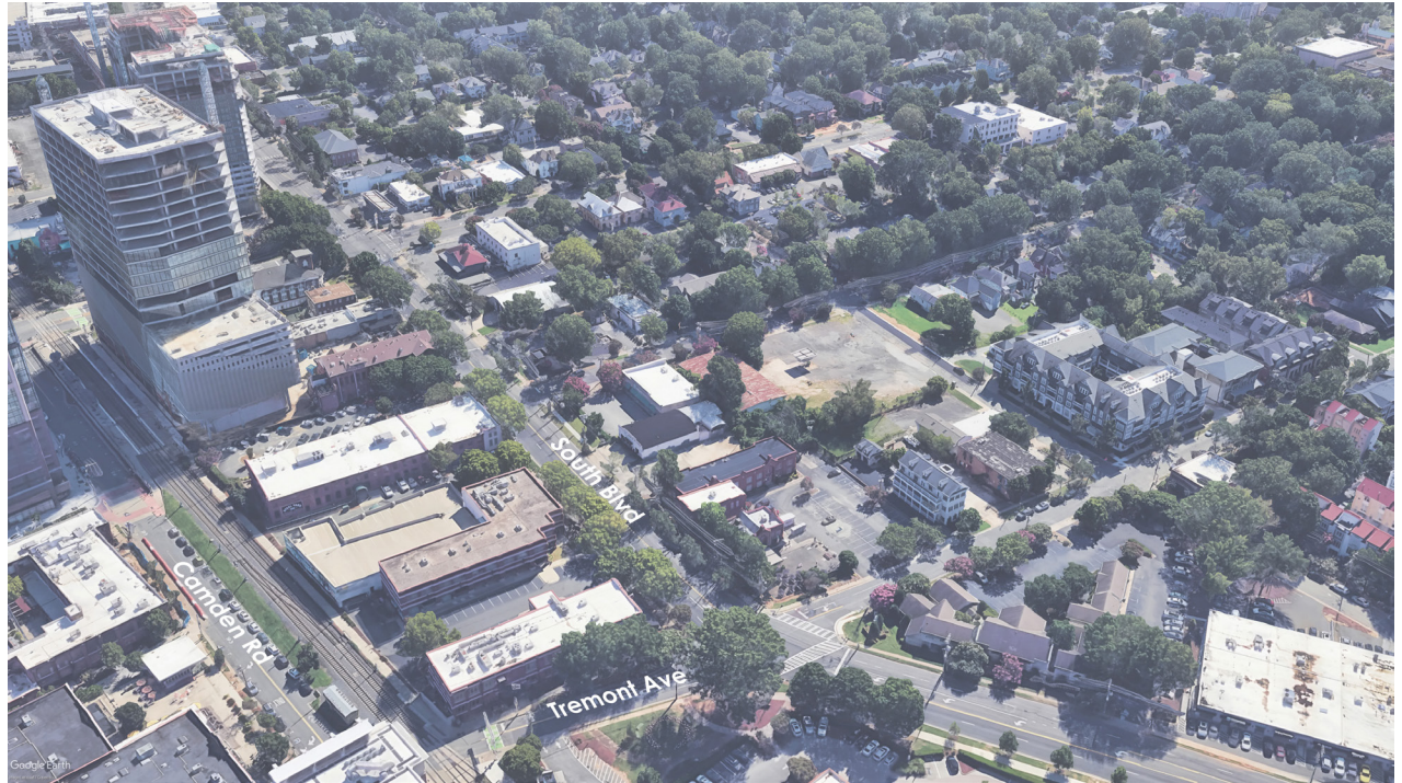
FIGURE 8: AERIAL OF EXISTING CONDITIONS
