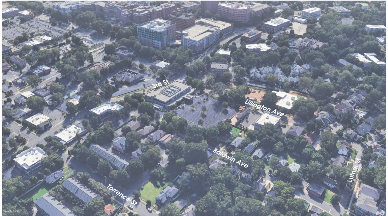
FIGURE 11: AERIAL OF EXISTING CONDITIONS
