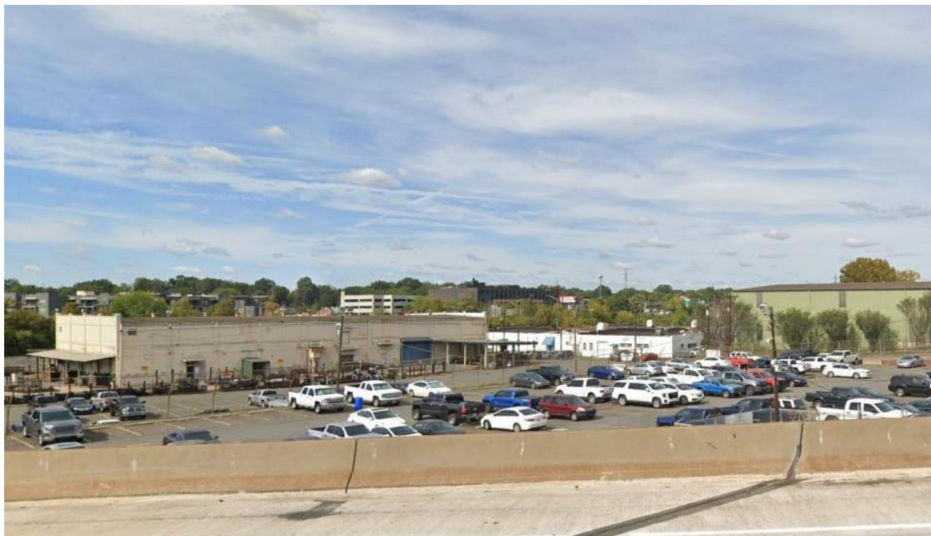
View of the site looking north from I-277 with parking, and warehousing for Charlotte Pipe and Foundry visible in the foreground.
