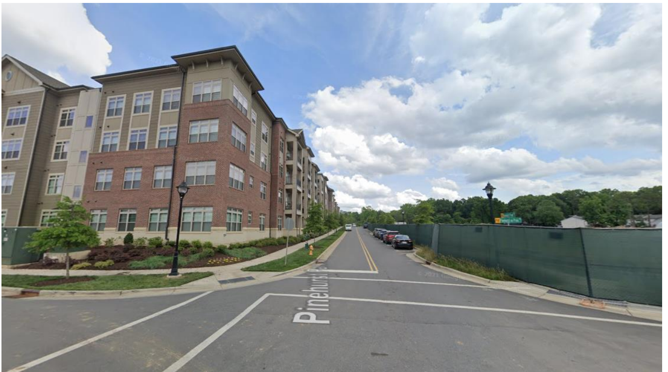
View of the site looking south from the intersection of Pinehurst on Providence Drive and Pinehurst Parkway. Building 3 in existing phase of the development is at the left of the image and Building 6 of the existing phase of the development is under construction at the right of the image.
