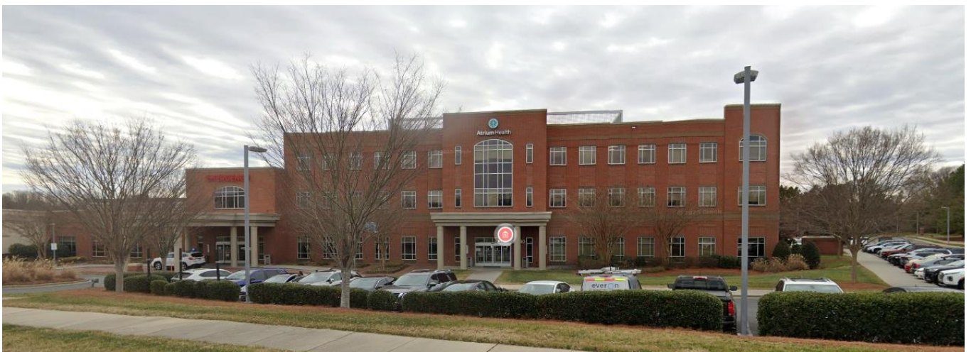
South of the site are medical offices.
