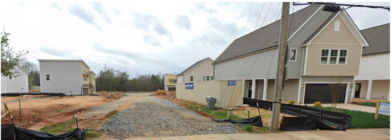
East of the site along Ervin Ln and Borgin Way are single family homes existing and under construction.
