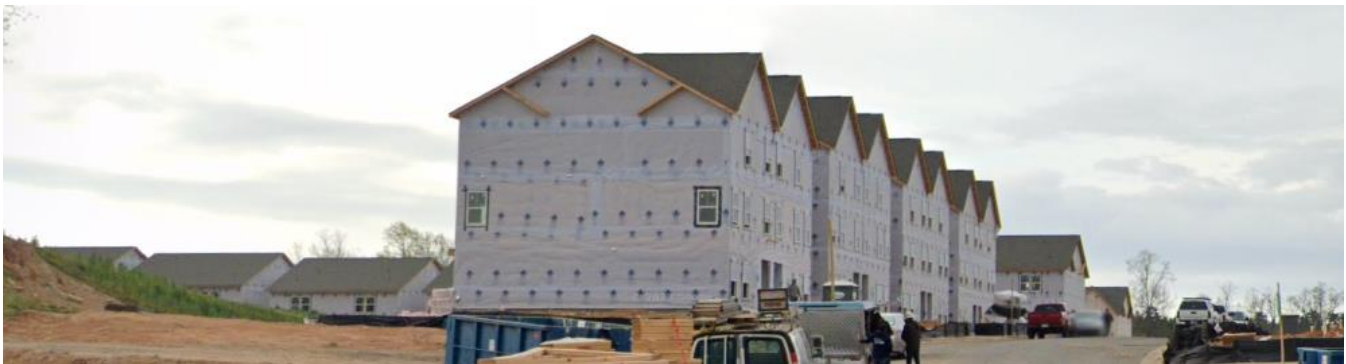
North of the site are single family attached and duplex dwellings under construction as Phases 2-4 of the Blu South development.
