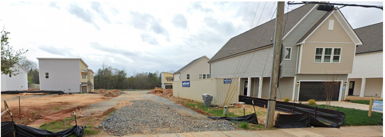
East of the site along Ervin Ln and Borgin Way are single family homes existing and under construction.
