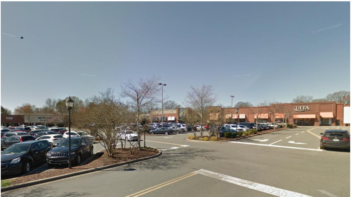
View north of the site of the Cotswold Village Shops development. The subject site is currently part of this development.
