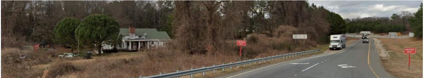
Street view of single-family residential use and the Interstate 485 ramp to the east of the site.
