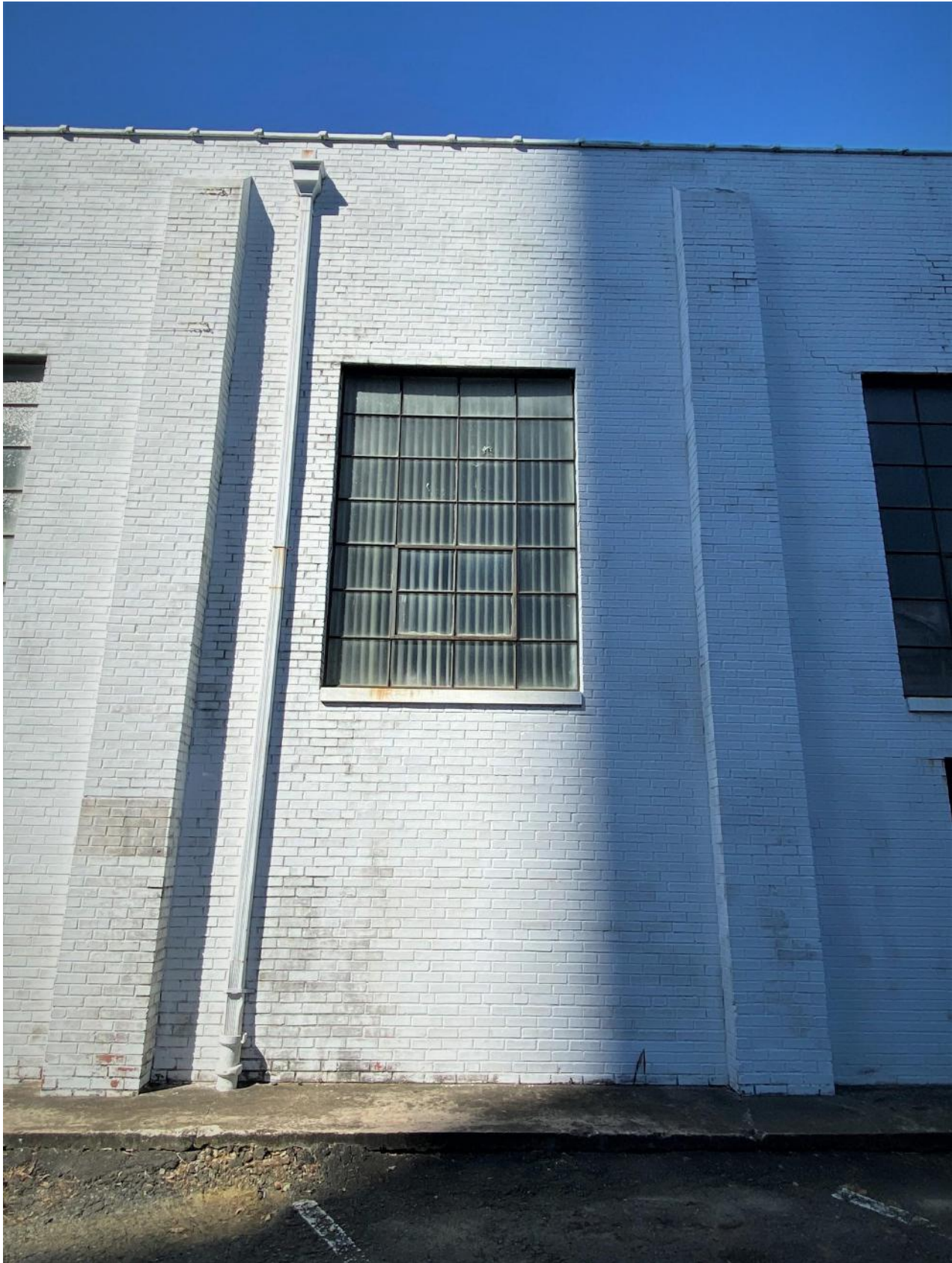
Fig. 10: Exterior Brick Columns
