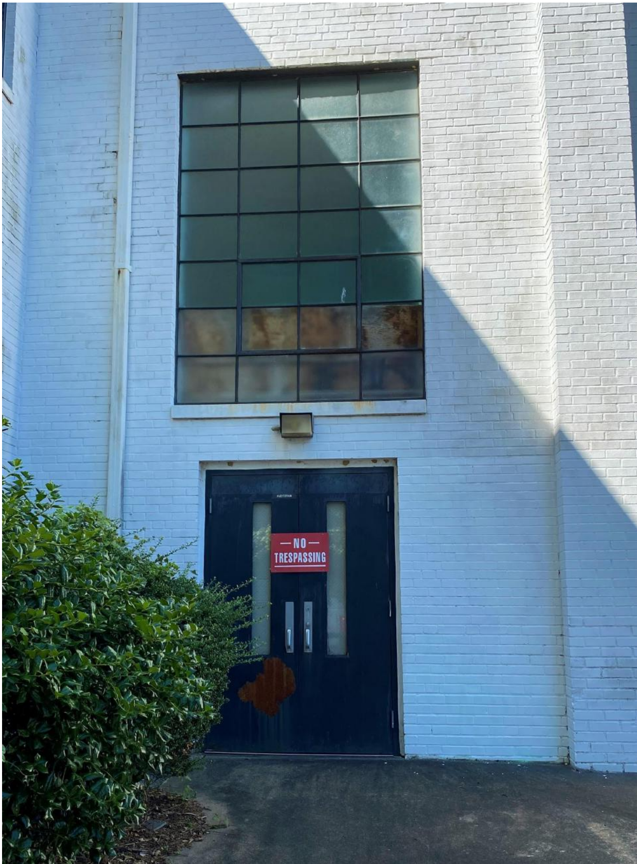
Fig. 12f: Side (East) Elevation Door
