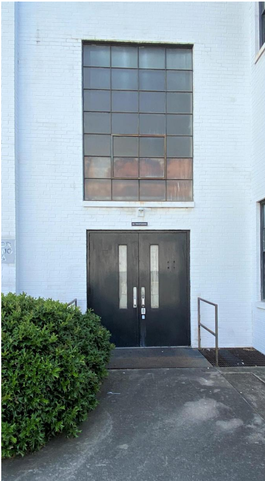
Fig. 11a: Four-over-seven Metal Framed Casement Windows
