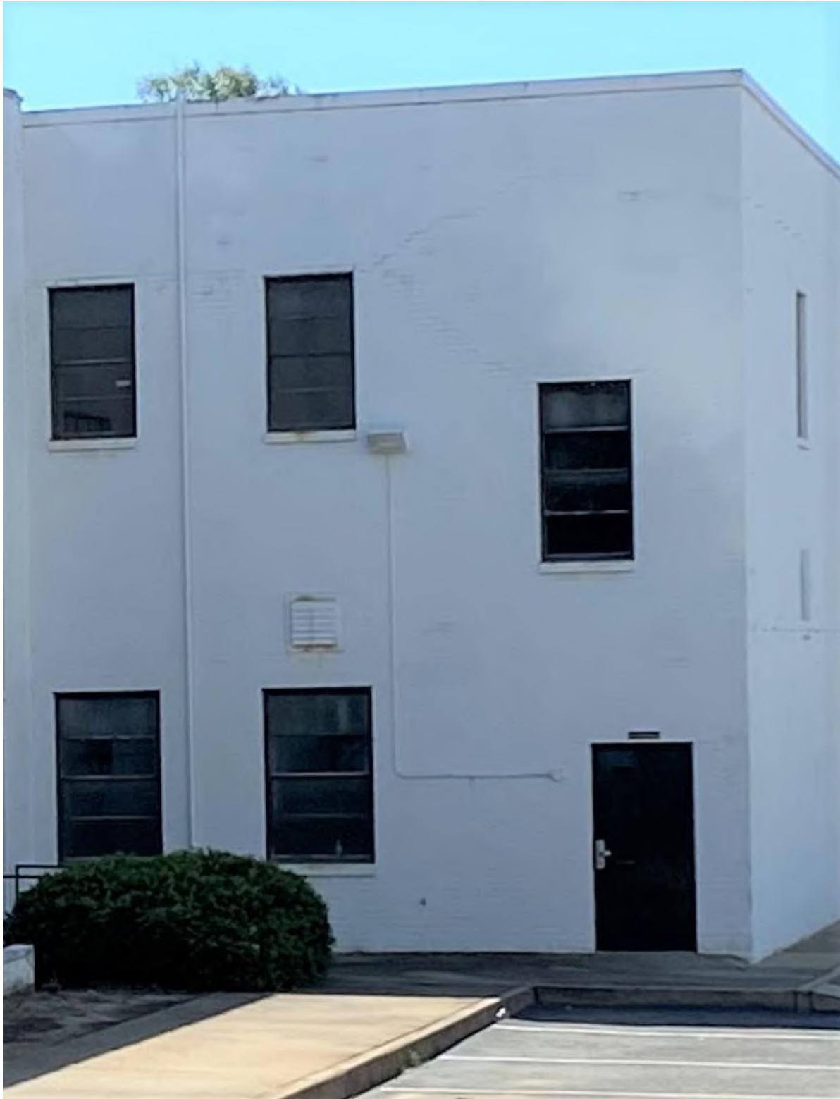
Fig. 11c: Two-over-two metal framed windows
