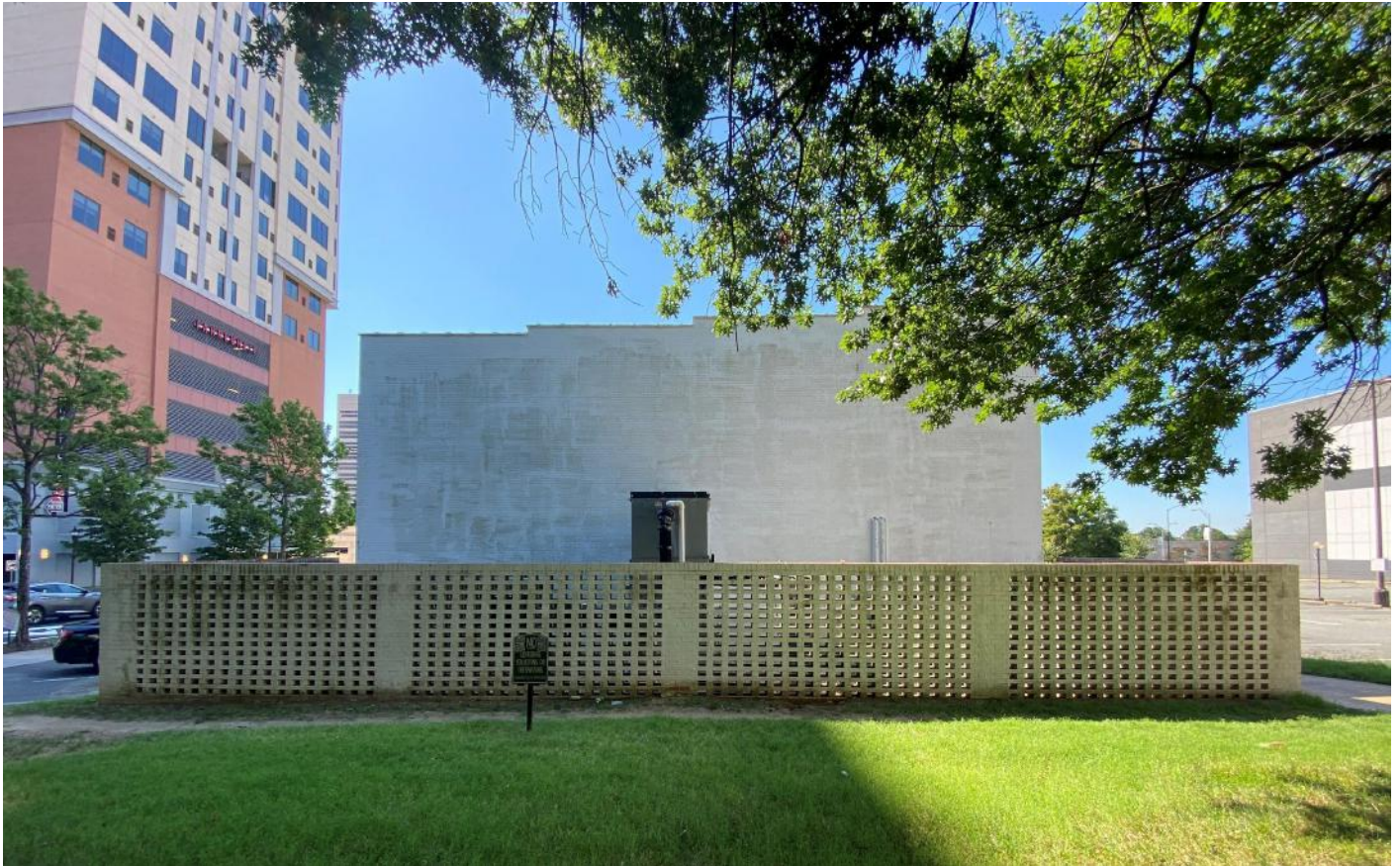
Fig. 7: Rear (Northeast) Elevation
