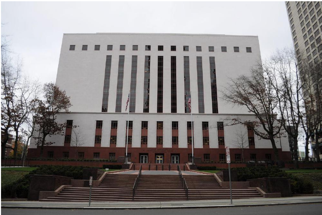
Old Federal Courthouse in Seattle, Washington
