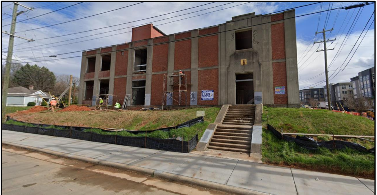
Looking SE toward the subject property along N. Brevard Street. Construction on this building has finished.
