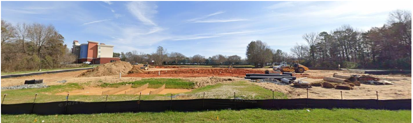
East of the site is development of a new hotel.
