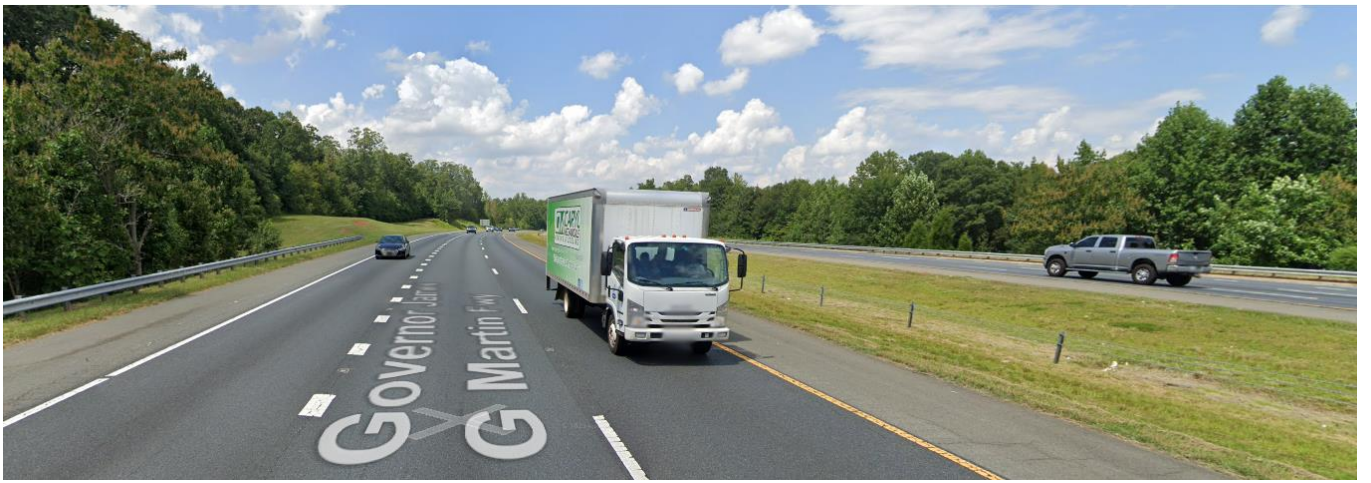
Interstate 485 borders the site to the east.
