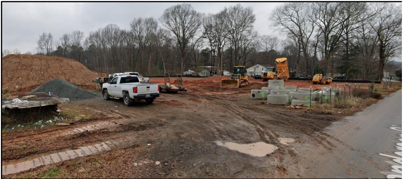
The property to the south is under construction with a single family subdivision.
