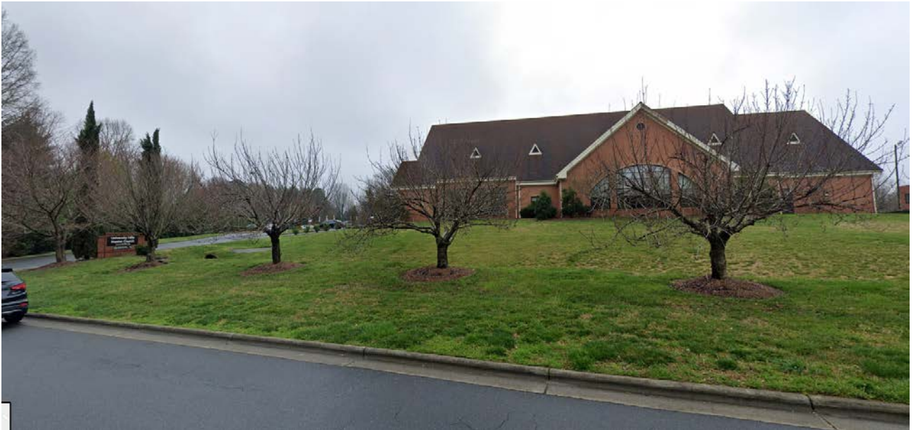
The property to the south is developed with a church.
