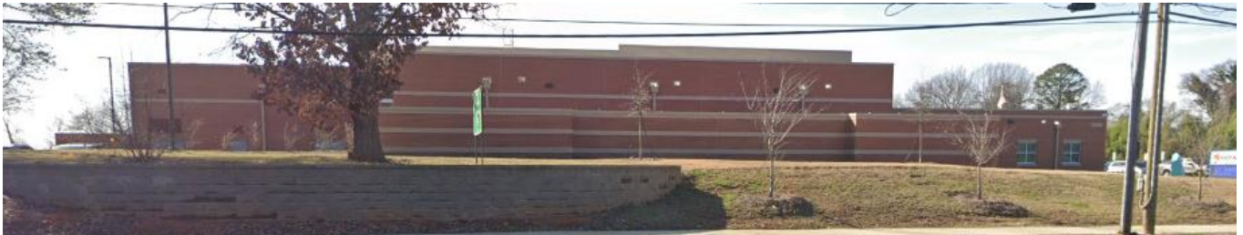
The property to the west of the site across Nations Ford Rd is developed with an institutional use.
