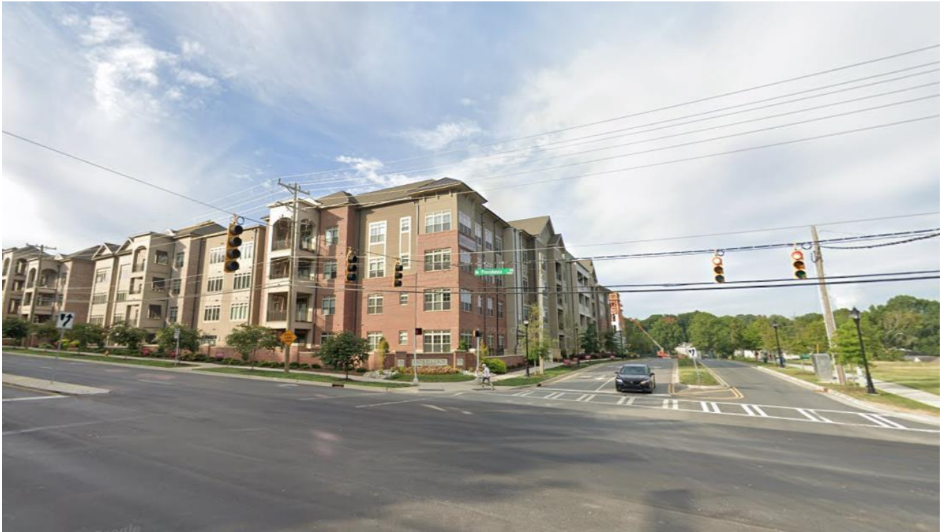
View of the site looking southwest from the intersection of Providence Road and Pinehurst on Providence Drive showing Building 3 in the existing phase of the development.
