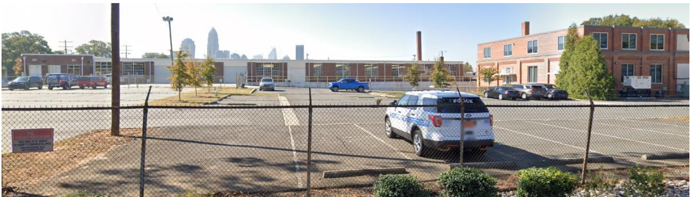
To the west of the site, is a Charlotte Fire Department office.
