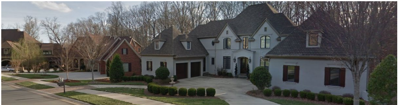
East of the portion of the site to be redeveloped are multi-family dwellings that are part of Legacy Arboretum Apartments that will remain. Beyond those east of the rezoning boundary are single family homes along Shadow Forest Dr.
