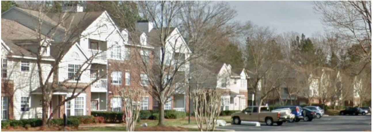
The site is developed with multi-family dwellings, part of Legacy Arboretum Apartments.
