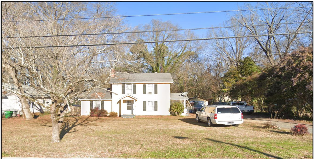
Subject site at 4019 Sofley.
