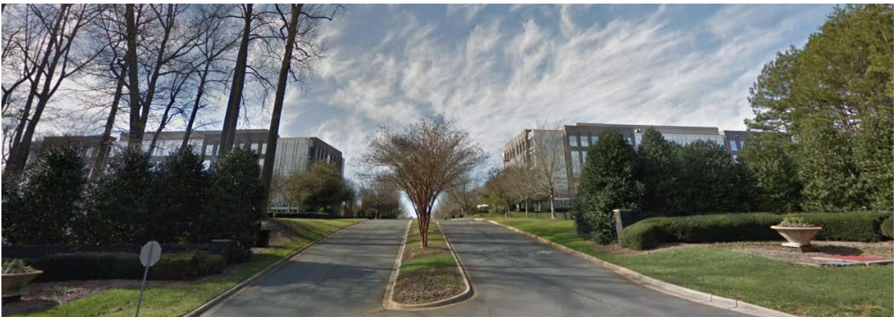
The adjacent properties to the east, south, and west are large research office parks.
